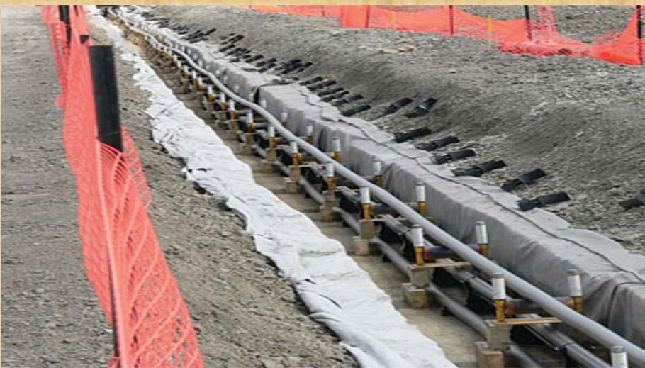
Underground cable installation process
