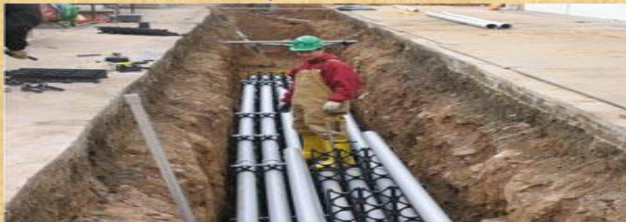
Underground cable installation process
